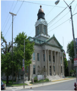
CRAWFORD COUNTY COURTHOUSE
