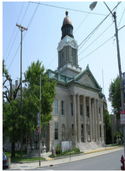
CRAWFORD COUNTY COURTHOUSE
