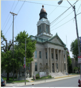
CRAWFORD COUNTY COURTHOUSE
