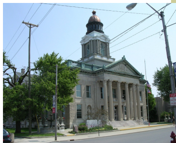
CRAWFORD COUNTY COURTHOUSE
