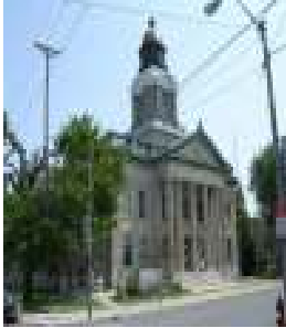
CRAWFORD COUNTY COURTHOUSE
